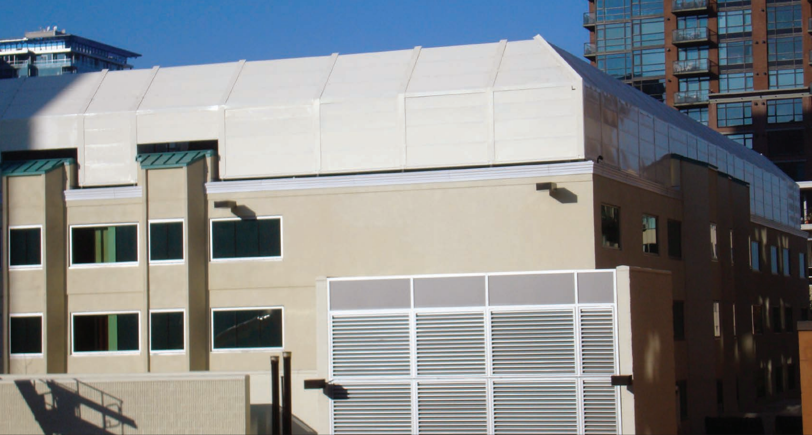
NOISEBLOCK™ wall system, Hospital Rooftop Equipment Yard
