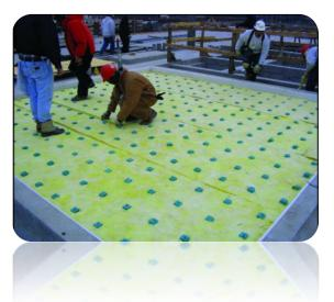
Moreover, the natural frequency of the KIP pad remains stable across a wide range of load scenarios, which is crucial for ensuring consistent noise control in environments where conditions may fluctuate. This performance predictability makes the system adaptable to many different project specifications and acoustic needs.
