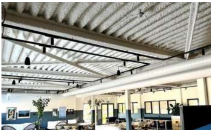
FIGURE 1: IMAGE OF ACOUSTIC SPRAY CLAD CEILING
