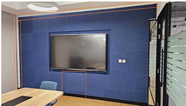
FIGURE 3: IMAGE SHOWING A RECENT PET PANEL INSTALLATION BY KINETICS
