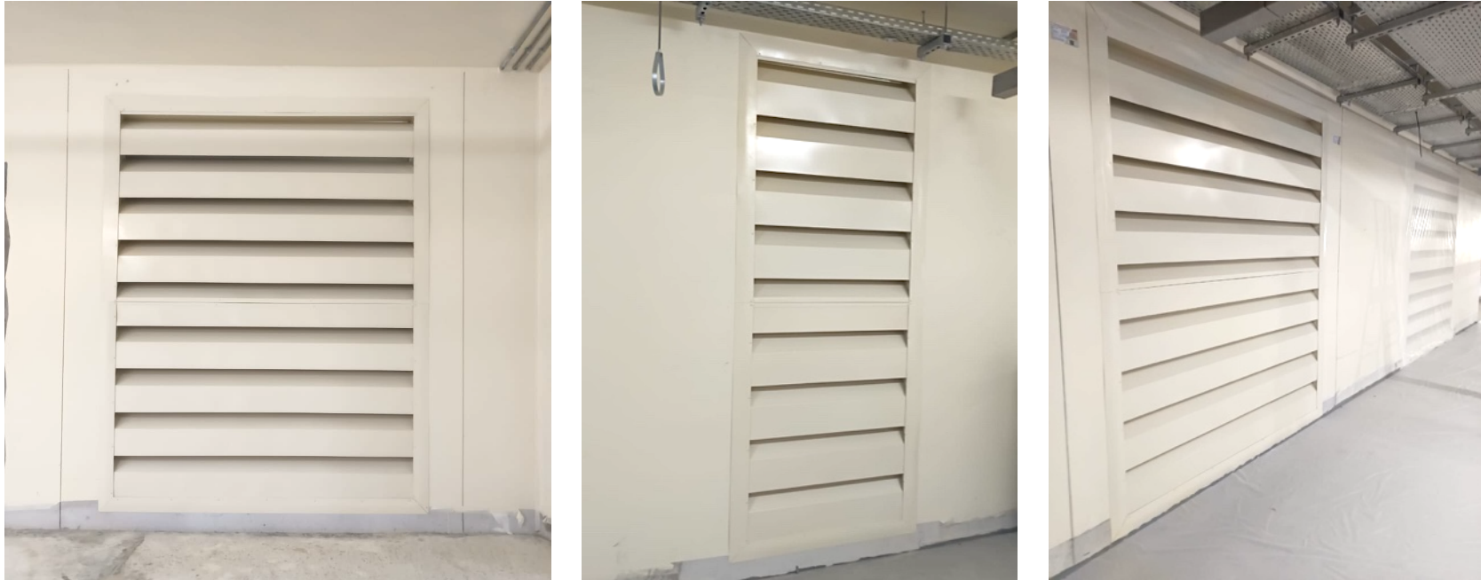
Installed 300mm Depth Double Bank Acoustic Louvers
