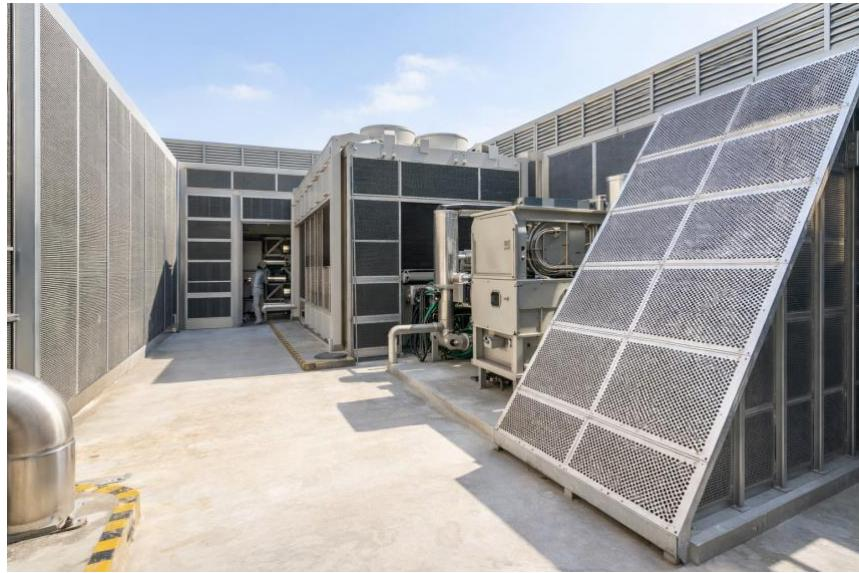
To achieve the required levels of noise and vibration control, a carefully engineered acoustic strategy was developed, addressing sound generation, propagation, and containment—while ensuring uninterrupted chiller operation and airflow performance.
